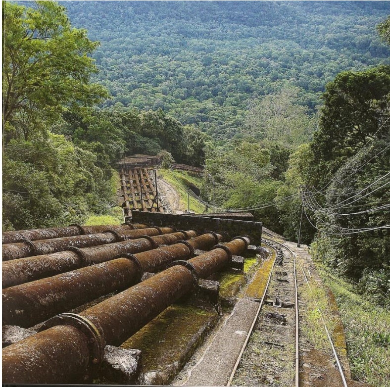
Cablecar track alongside pipelines from water chamber to plant
