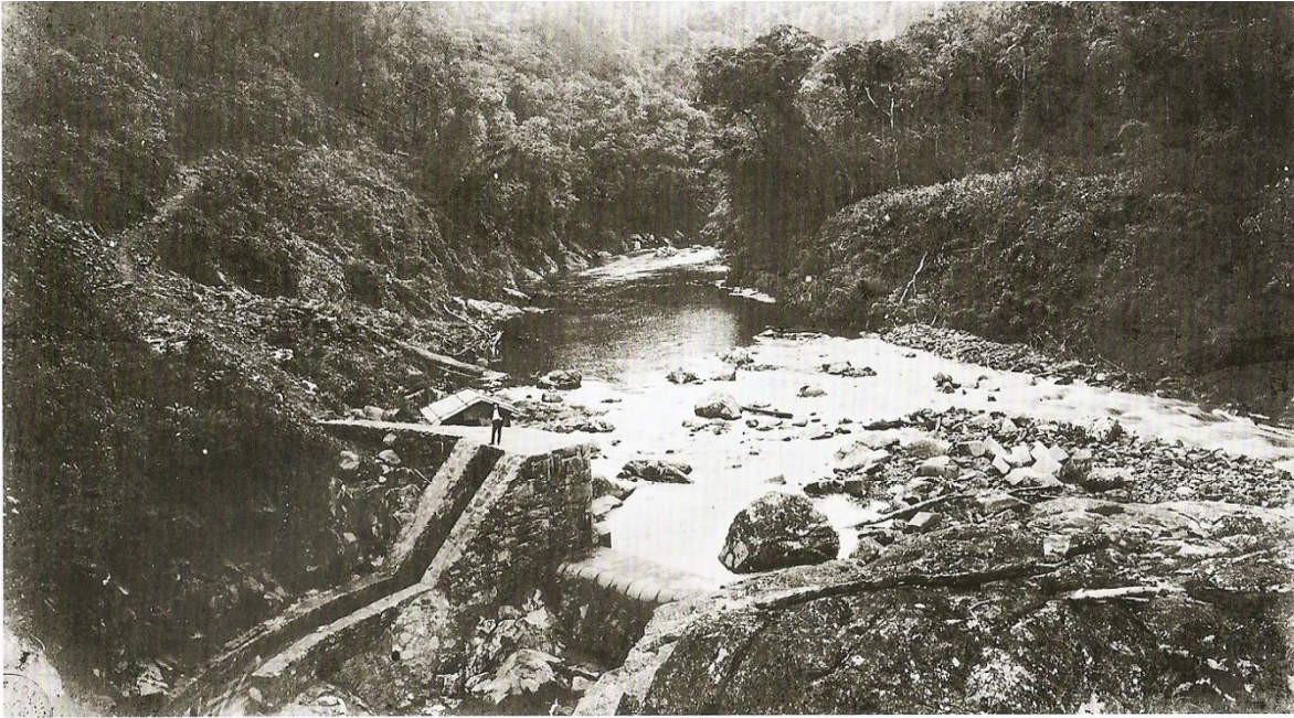
Construction of the dam around 1905-6
