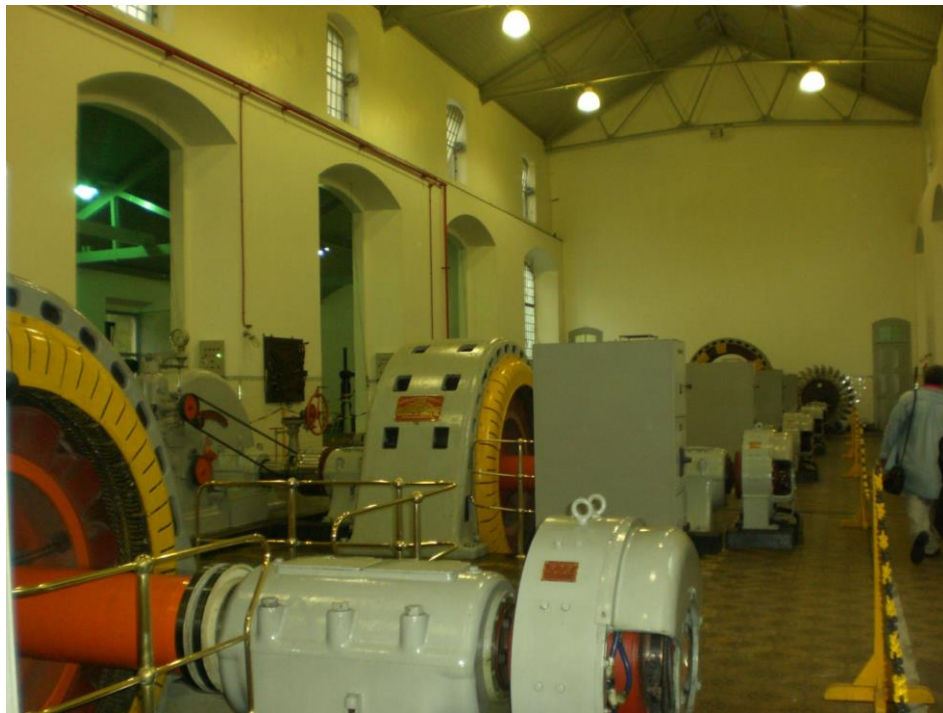
Turbine and generator room in use since 1910
