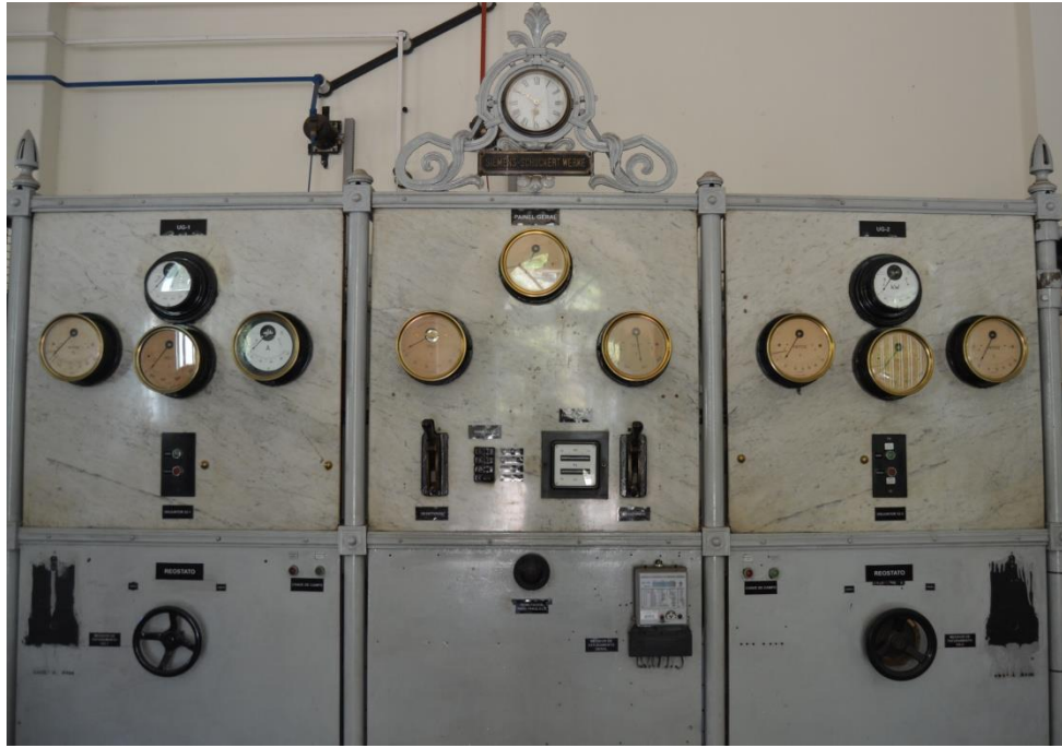
Santa Alice. Painel de controle (1907)
